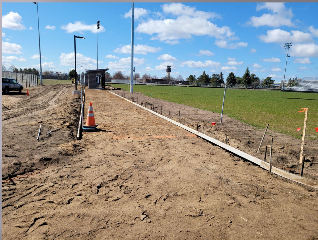
Concrete work around soccer fields, scorers booth and varsity dugout.
