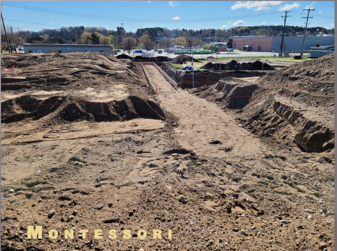
Concrete footings and foundation prep work for the gym.
