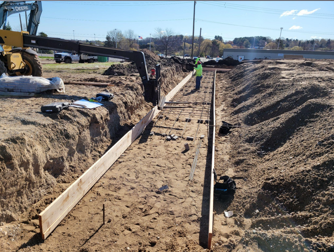
Concrete footings and foundation prep work for the gym.
