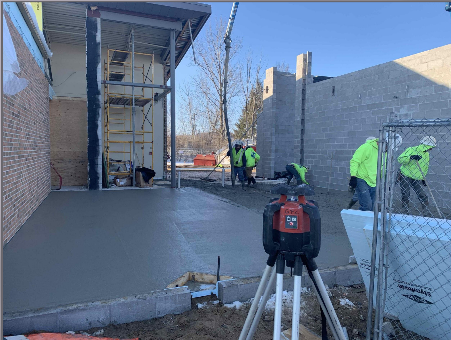
New slab being poured.
