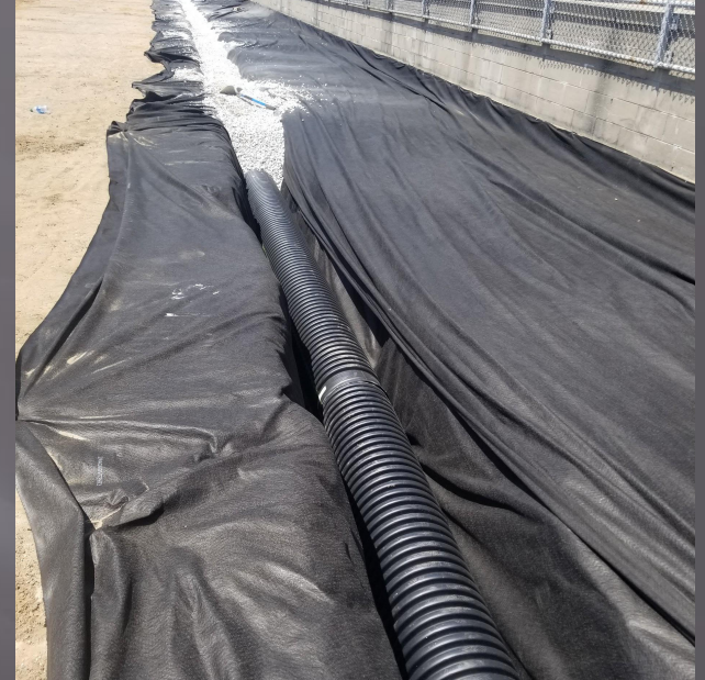
A portion of the new under-drain system going in.
