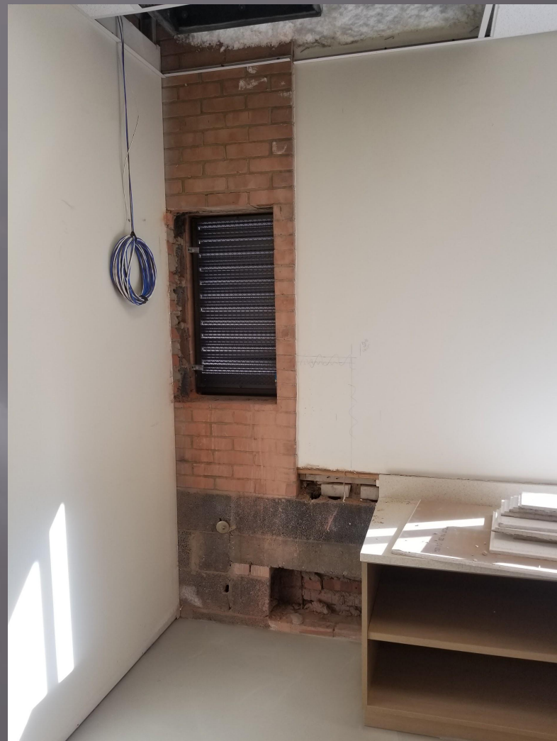
Typical classroom renovations.
