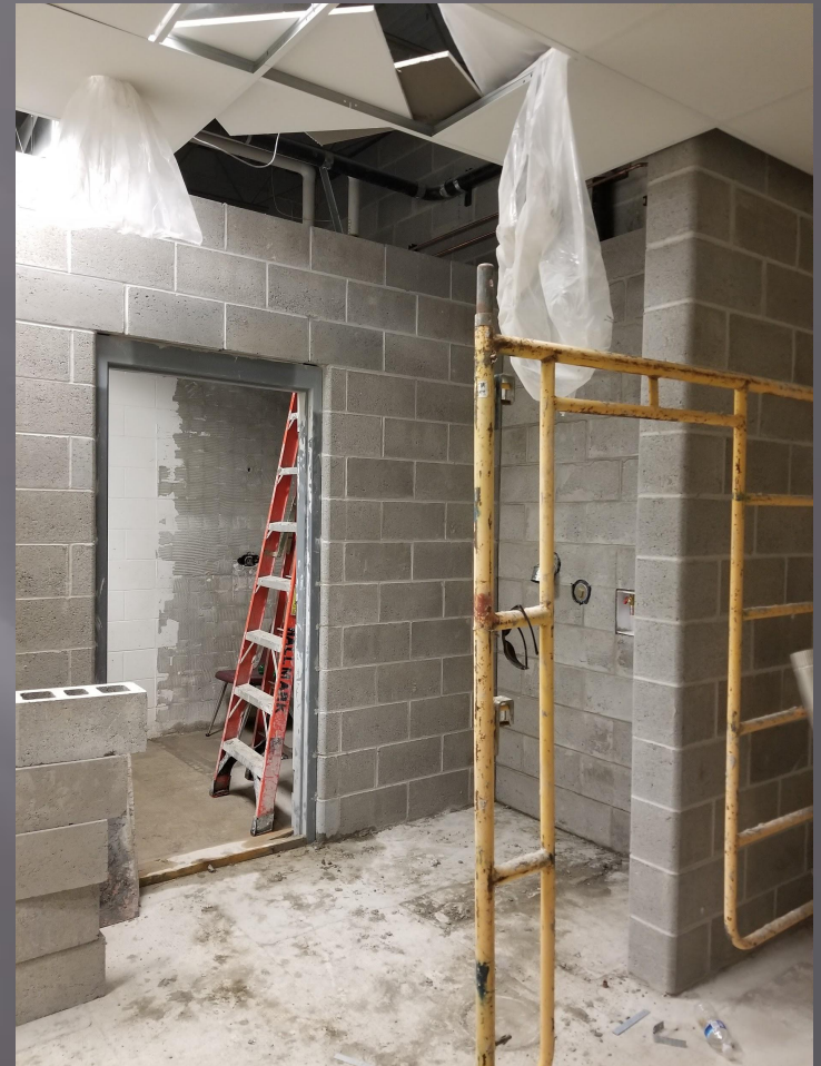
Main Office and single user restroom/shower/laundry
