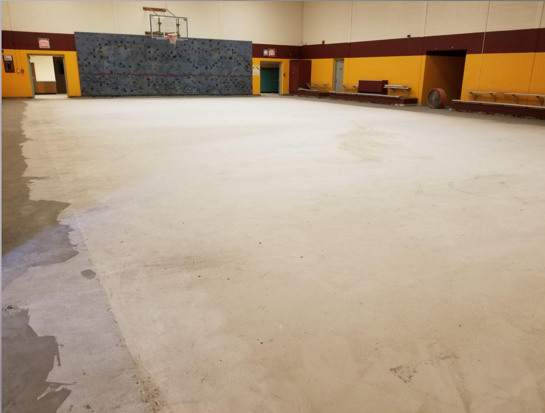
Floor leveling, next step new flooring installation.
